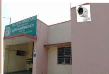
Surveillance Camera at COA, Kota
