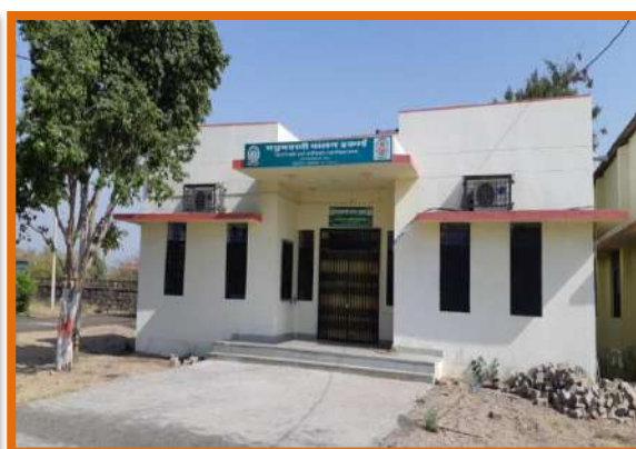
Building of Honey Processing Unit
