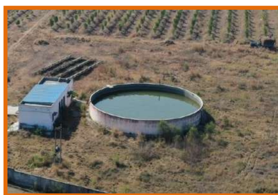
Water Harvesting Tank
