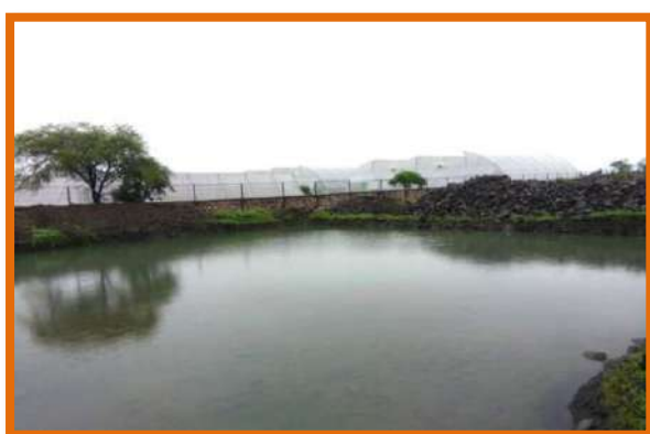
Plastic line water Rain Water Harvesting Pond
